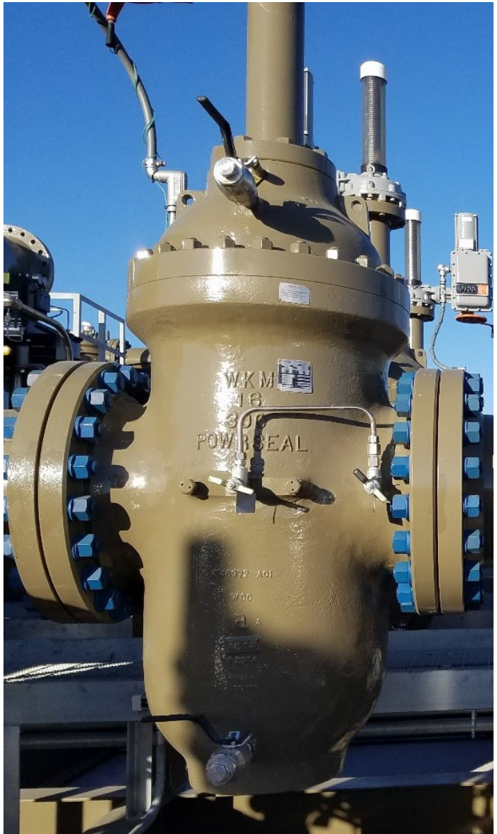
16-in, Class 300 Pow-R-Seal valve.
